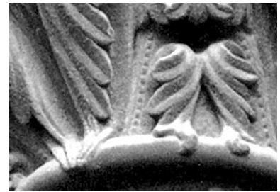
Saint-Denis west portal W.sR1 detail
