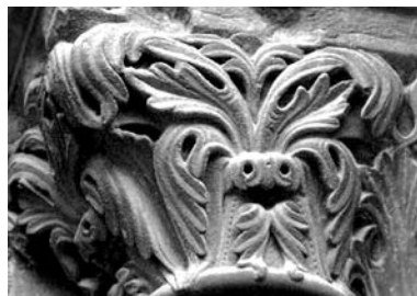
Saint-Denis west portal W.sR1 1132
